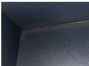
Insufficient coating thickness in inner edges
